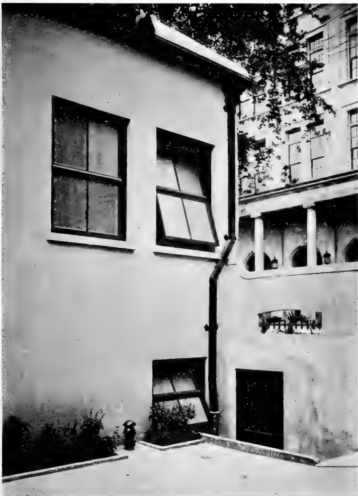
The Court Showing the Wall, and Fence Wall Built of Reinforced Concrete
